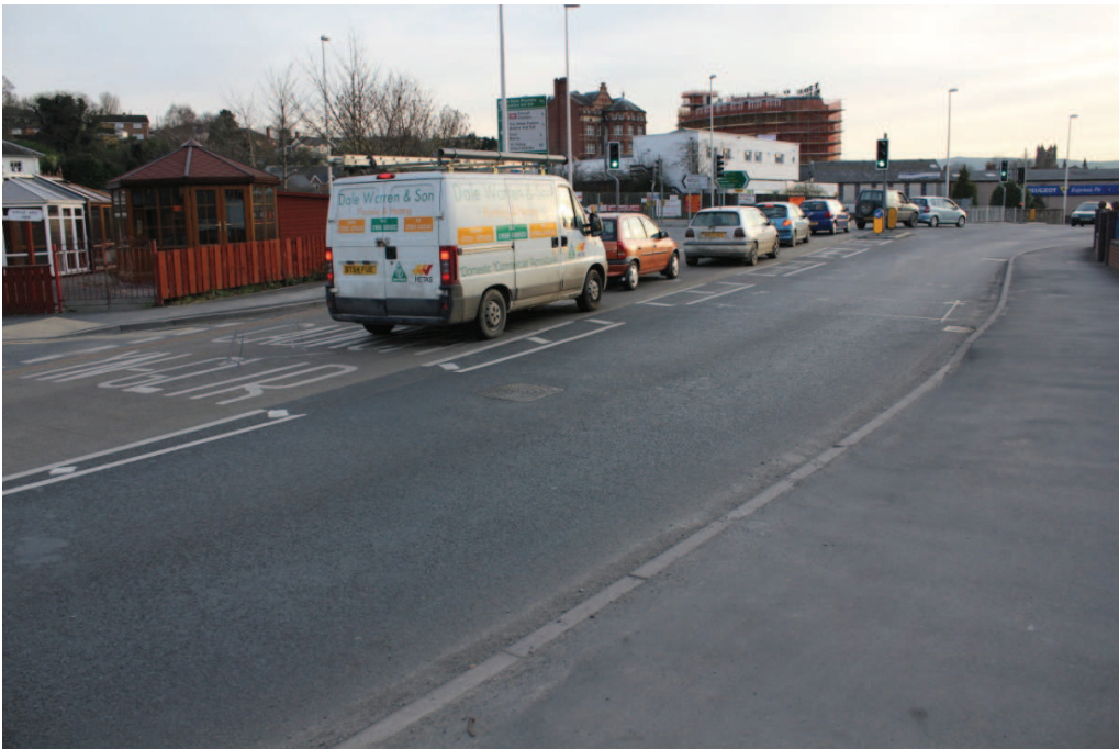
Photograph 3.2: Showing the right turn lane and the ‘keep clear’ markings over Sheaf Street.
